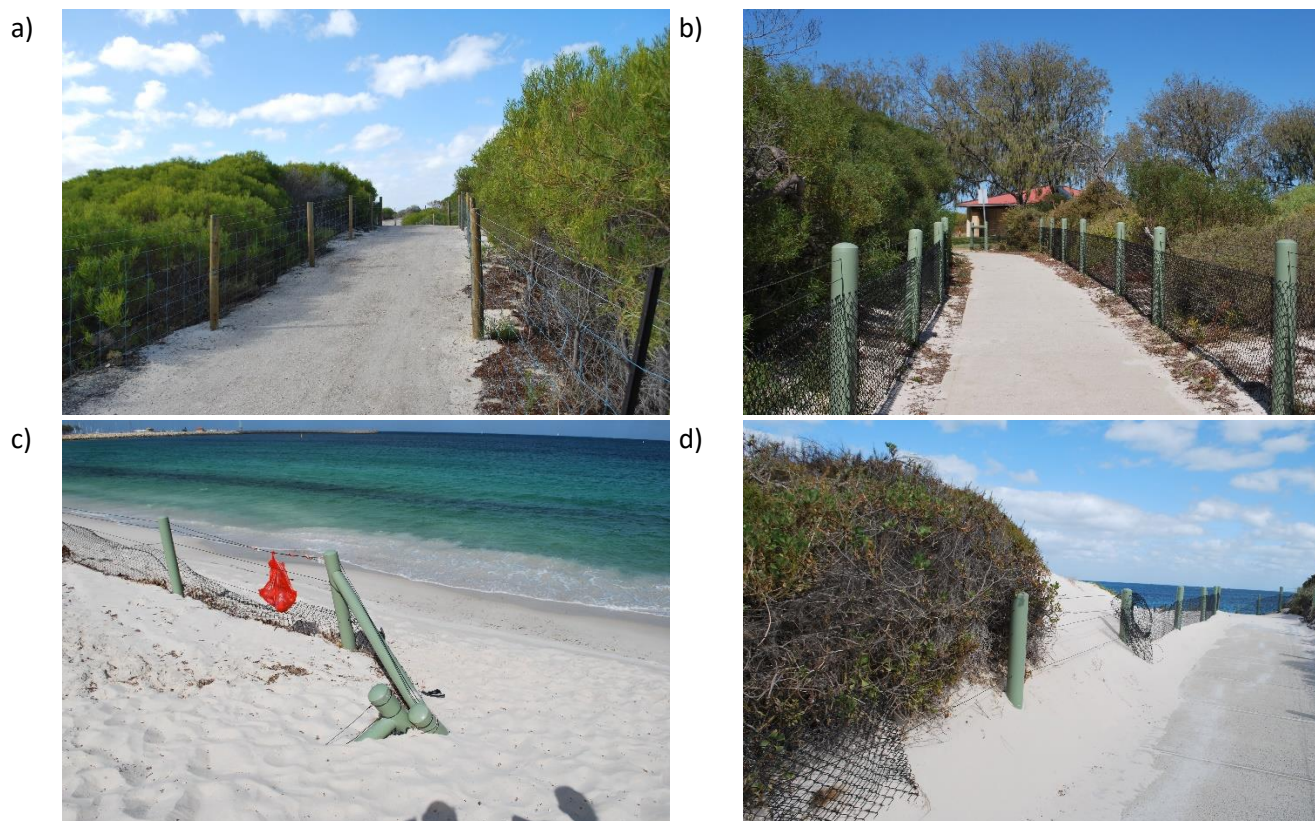
Figure 20: Fencing: a) pine post and square ringlock and wire fencing, b) PVC sleeves over pine posts and chainmesh fencing, c) fencing buried due to coastal erosion of sand dunes, d) fencing damaged along beach access path.
