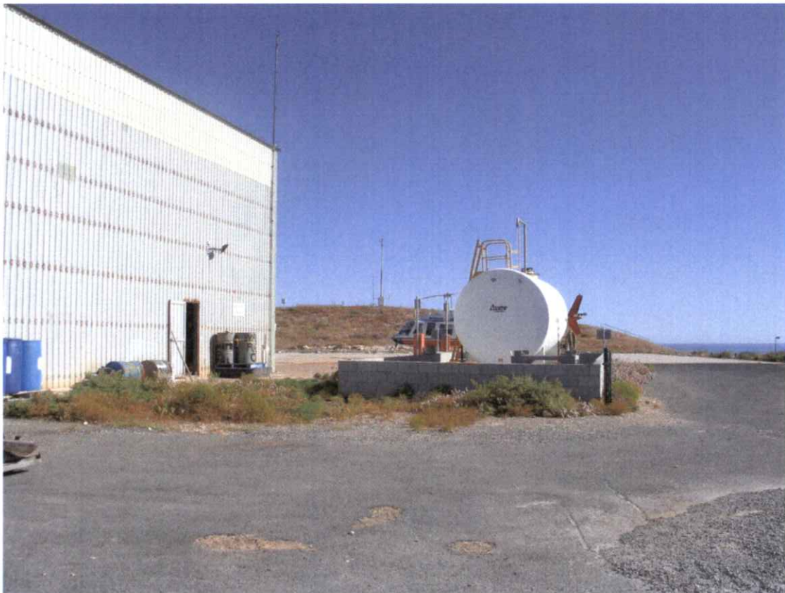
Photo 4. Vegetation around the helicopter Jet Fuel tanks.
