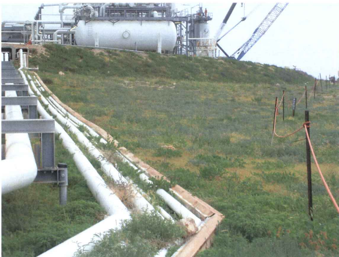
Photo 1. Vegetation under pipelines and cable trays.
